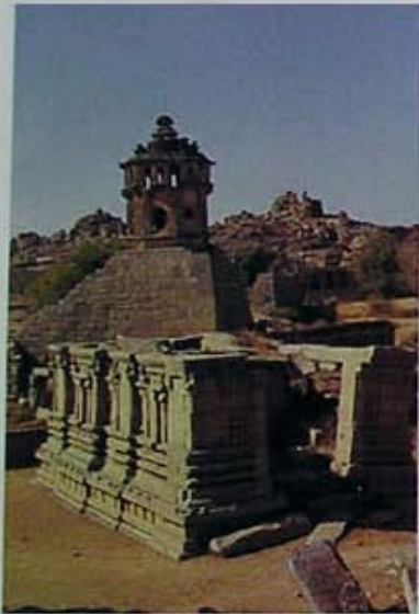
A small dilapidated temple, called the Madhava temple with the octagonal watchtower in the background.
