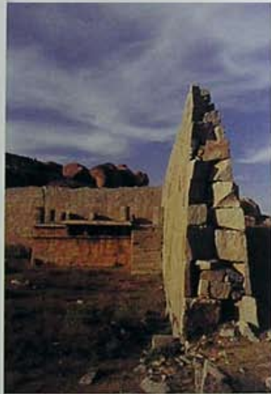
High enclosure walls of the royal centre. Note the cross-section of the tapering wall in which blocks of stone are dexterously laid without any cementing material.
