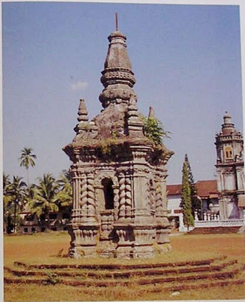
Cross at St. Alex Church, Kurltor, and in the piazza fronting Espírito Santo, Holy Spirit Church (facing page) at Margao. The Goan artisan showed off, in these "bits" of stucco moulding, all the decorative devices—baroque curves, rococo volutes and twisted columns—which he had employed while shaping church interiors. The Portuguese architect provided the general stylistic scheme.
